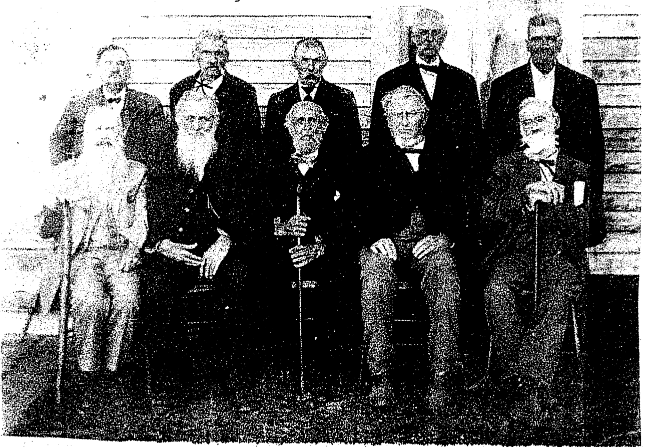
Masonic Temple on Water Street. Front row, left to right: C.H. Sexton, Joseph Bland , L.D. Spencer, A.B. Lyons, and Sam Levingston, Sr. Back Row, left to right: Dr. Sanders, W.D. Street, Dan Morrison, A. McKay, and W.R. Bolin. This lodge building was erected on land purchased in 1878 and was the second one in Orange owned by Madison Lodge No. 126, the first structure (built in 1854 and also on Water Street) having been destroyed in the great storm of 1865 which almost wiped out Orange. The building pictured was on Water Street between Henderson and Division streets. The third, or present, temple, on the corner of Elm and fifth streets, was first occupied in 1926.
